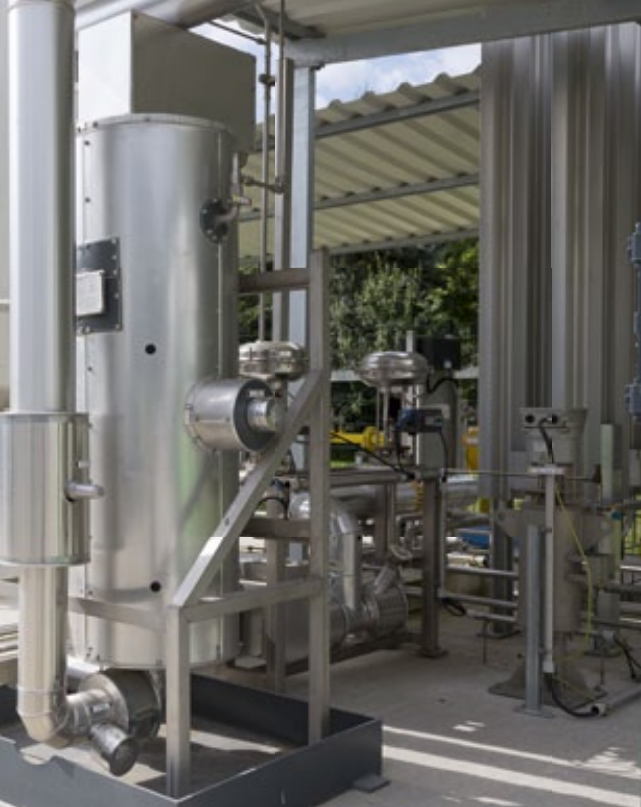
Cold exchanger within the LNG system
