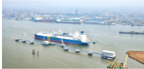
Klaipeda LNG terminal based on FSRU Independence
