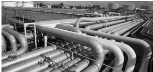
State fuel reserves terminal
