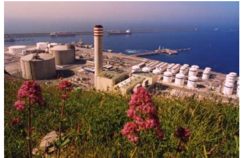
BBG regasification terminal and BBE CCGT power plant. Bilbao
