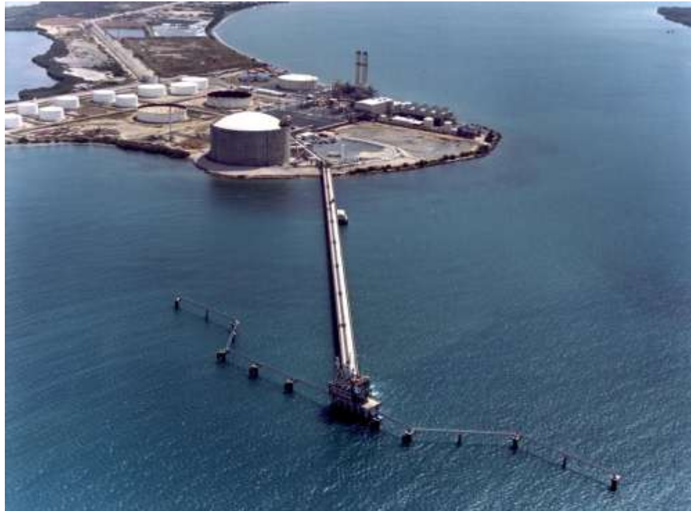
ECOELECTRICA regasification terminal and power plant. Puerto Rico
